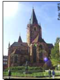
Heavy old building
